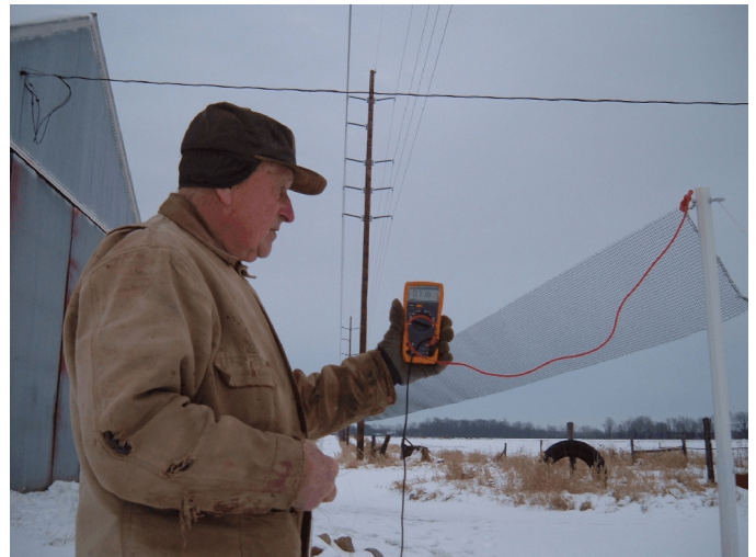
Mr. Chick Reading 71.6 Volts under 46 kV Transmission Line
